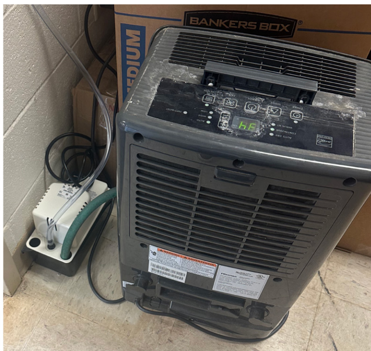
Right: Dehumidifier in the Greenville County circuit court clerk's office storage area, with a hose from the reservoir draining the water into a dehumidifier pump, then up through the ceiling tiles, and then outside.
