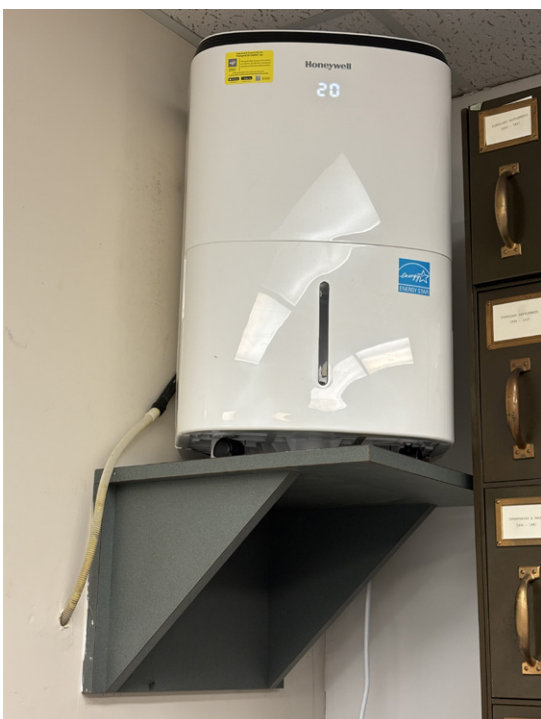
Left: Dehumidifier mounted on an elevated platform in the Craig County circuit court clerk's office records room, with a hose from the reservoir draining the water outside.
